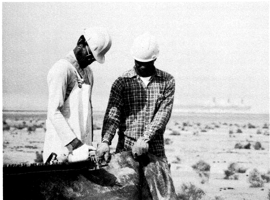
Figure 2. Superior strength of seam allows seams to be stressed during installation.
