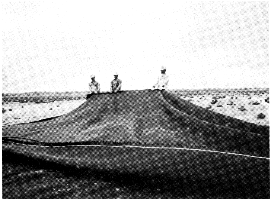
Figure 1. On site seaming of a geotextile using Kevlar® aramid, TEX 420.
